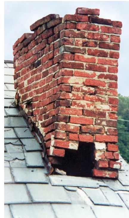
[7 a-b] This crumbling chimney was restored to its historic appearance using matching bricks.
