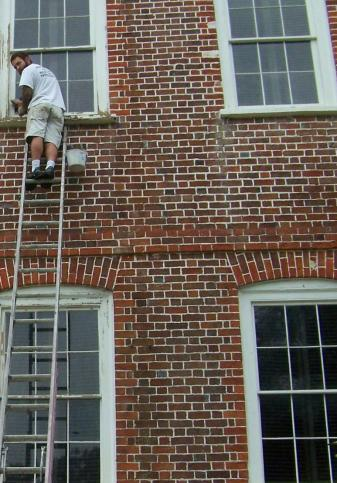
Note: Avoid Damaging Treatments. Example: Sandblasting of Brick is Frequently Proposed, Which can Cause Significant Damage to Historic Building Material. The Cleaning of Structures, if Appropriate, Should be Undertaken Using the Gentlest Means Possible.
