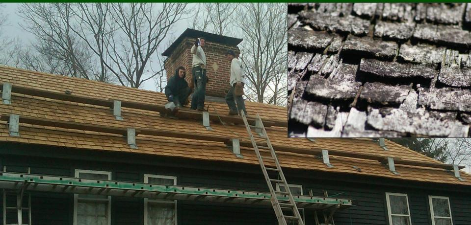
Many Times, Historic Fabric has Deteriorated Beyond Repair. This Often Includes Woodwork, Windows, Roofs & etc. When the Severity of Deterioration Requires Replacement of a Distinctive Feature, the New Feature Should Match the Old in Design, Color, Texture, & Other Visual Qualities, and, Where Possible, Materials
