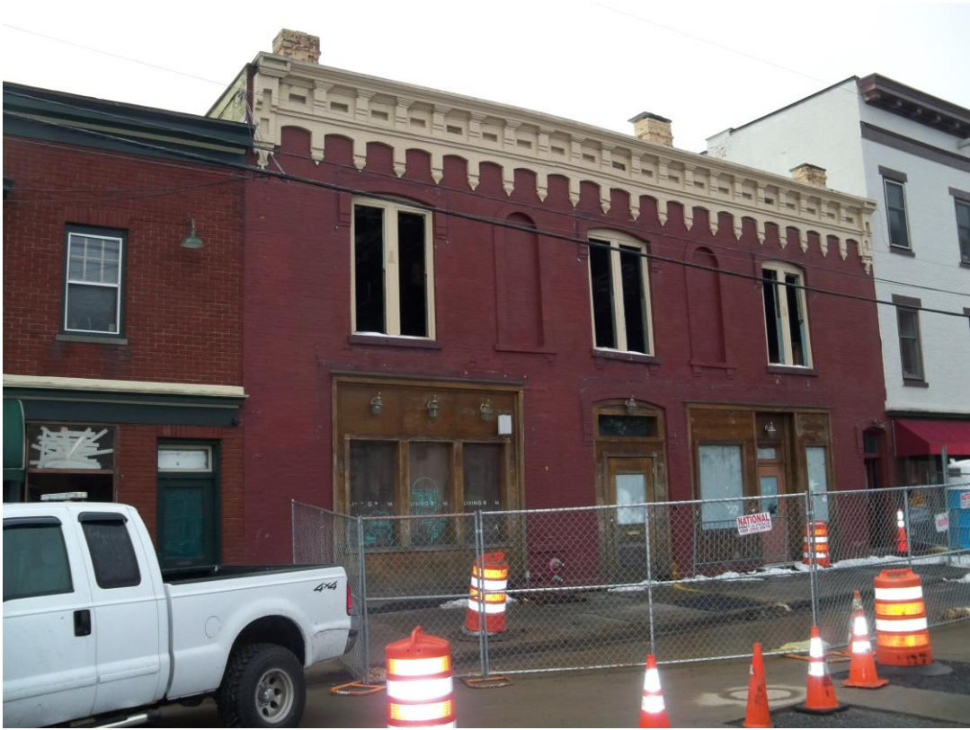
Photograph 1 - front masonry façade looking southwest.
