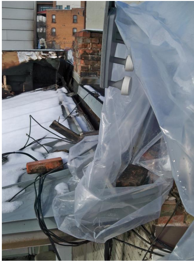
Photograph 3 - separation gap between rear building wall and rear stairwell.
