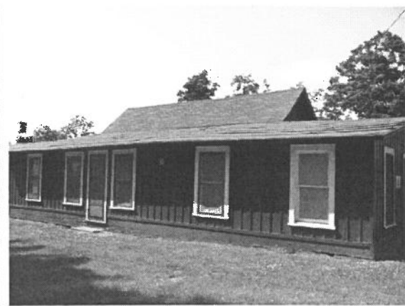
BH43 with L-shaped addition. Addition with its low sloped roof has a rolled asphalt cladding which is lifted and curling.
