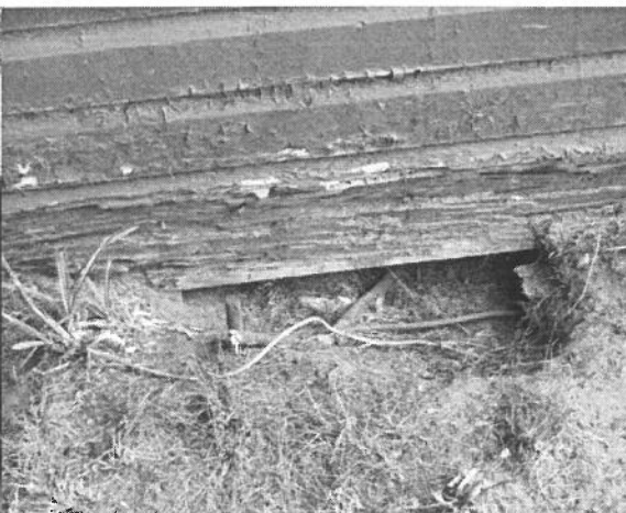
Typical rot at sill and lower clapboard courses on BH53.
