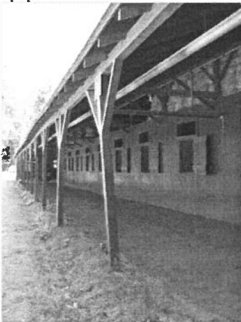
Rear shed row of Barn #30 illustrating shuttered screen windows and upper transom. Note also the shed post that is out of plumb.
