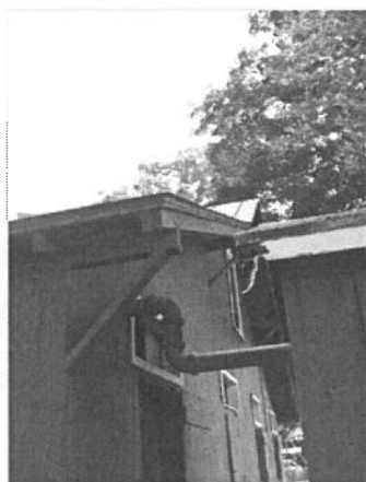
Connection between Barn and Sprinkler valve house.
