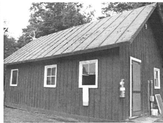
BH59 illustrates some of the worst conditions relating to the metal roofs, the windows and rotted or missing battens.
