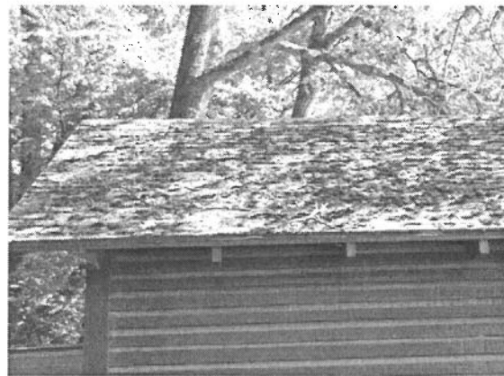
Asphalt roof on BH49 is covered with moss on north slope.
